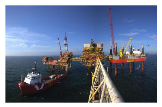
The Seafox 4 currently is contracted by ONEgas and stands alongside the Leman Alpha AC jacket to deliver accommodation and hook-up services.
